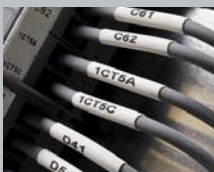
Wire & Cable Labeling
