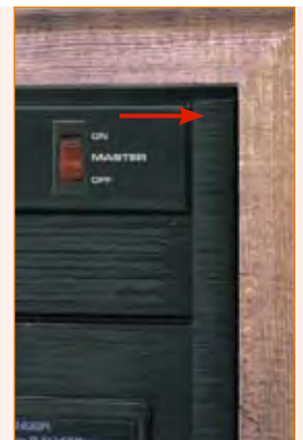
with trim strip installed
