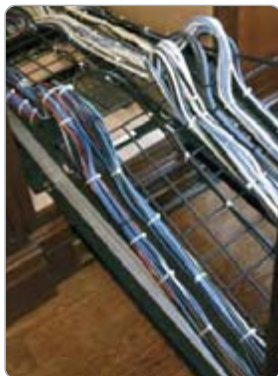
AXS-WT50 cable management tray recommended for high cable density installations
