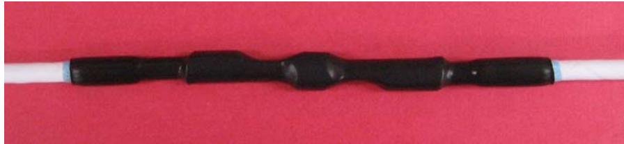
Picture 2. Installed RT-555 sealing sleeve on splices
