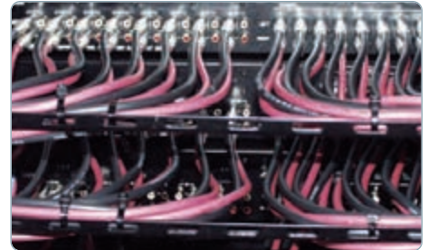
an example of proper cable management using the LBP-1A lacer bar, provided by Dave Zastrow - Multimedia Solutions
