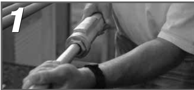
Slide the fitting onto the conduit until it stops at the internal sliding bushing. Tighten and you're ready. No parts to reassemble!
