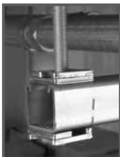
New method using Trapnut® Strut Fastener
