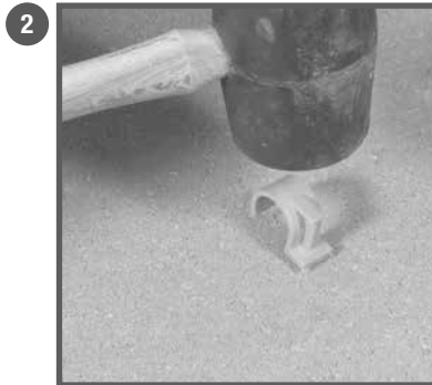
2 Tap clamp with hammer until fully inserted.
