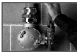
5. Install hub on enclosure
