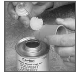
Apply a uniform coat of cement.
