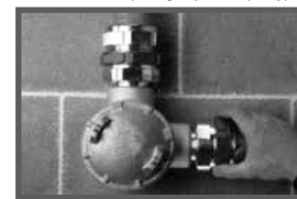
6. Insert cable and tighten red union
