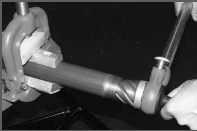
Ream the conduit with approved reamers. Spiral and straight-style reamers are both acceptable.
