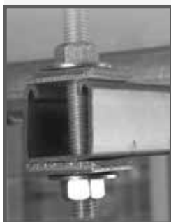
Standard method using nuts and washers
