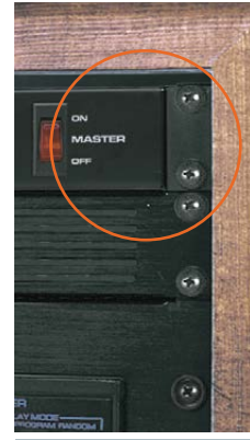
without trim strip installed
